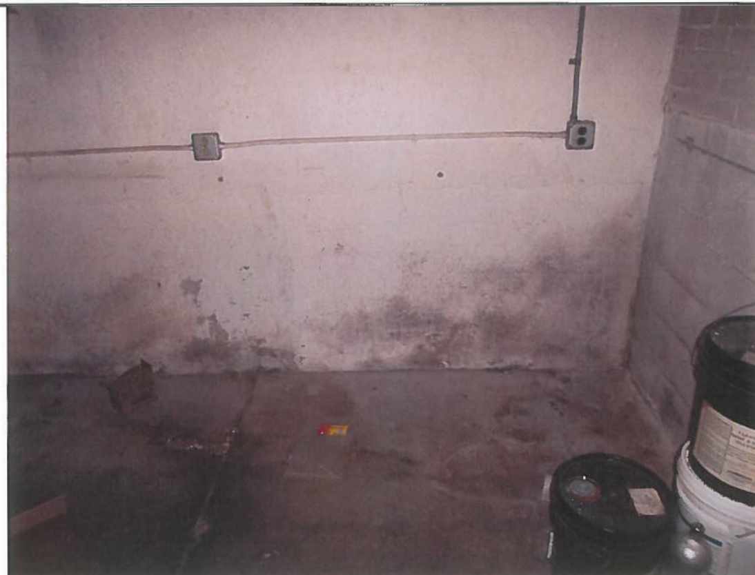
Basement – Suspect visible mold growth on west concrete wall (on paint) of Fire Department Storage Room.
