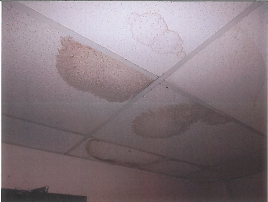
1 st Floor – Water stained ceiling tiles within the Roll Call area of the Police Department.
