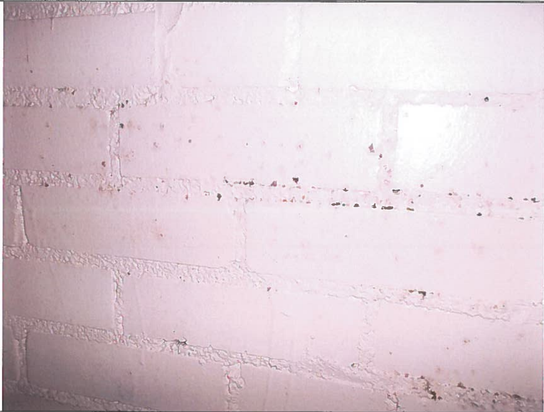
2 nd Floor - Suspect visible mold growth and visible water on north brick wall (on paint) of Ms. Price's Office.
