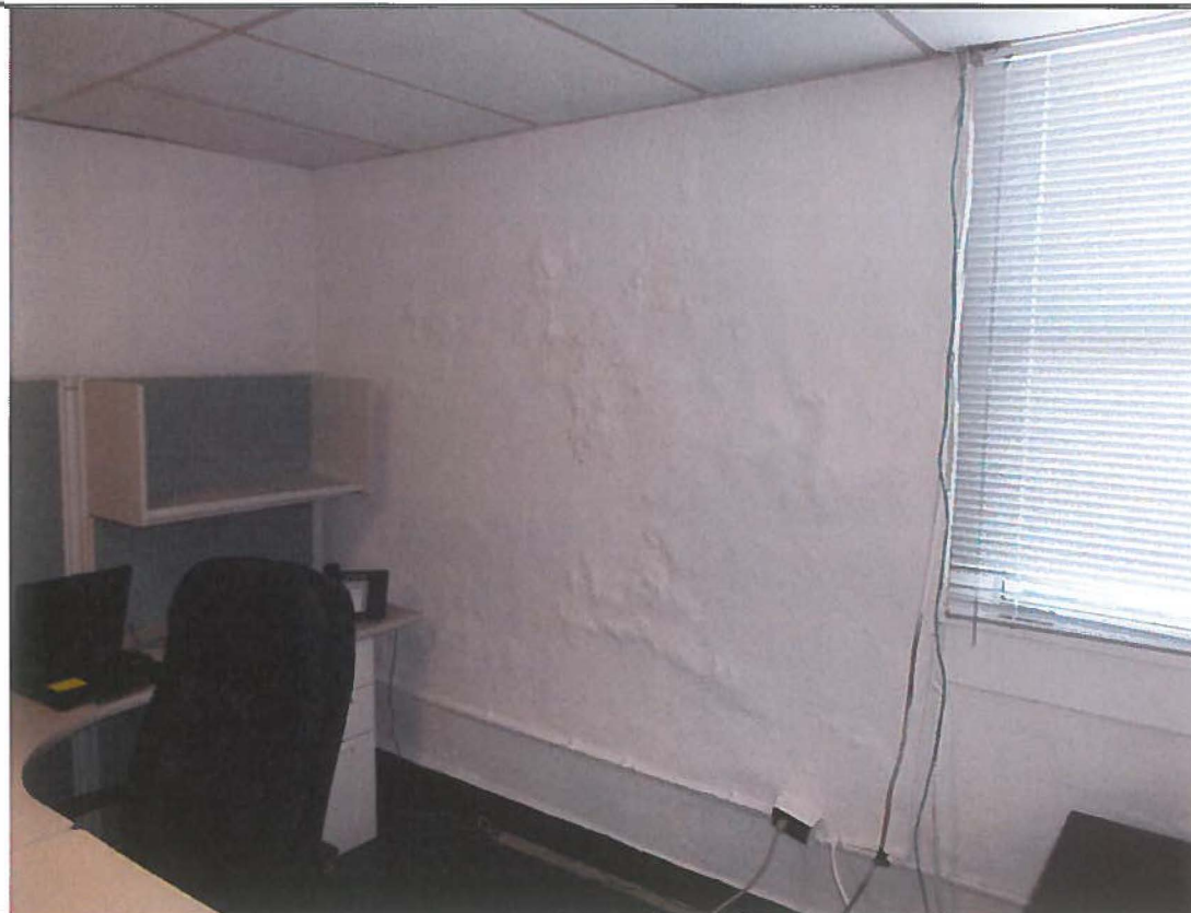
3 rd Floor – Water damage on east plaster wall in D.A.R.E. office.
