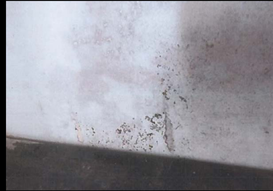
3 RD FLOOR SUSPECT VISIBLE MOLD GROWTH WEST PLASTER WALL-COMMAND CENTER
