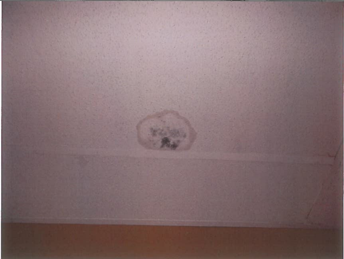
1 st Floor – Suspect visible mold and water staining on ceiling tiles within the Fire Chief's Office.
