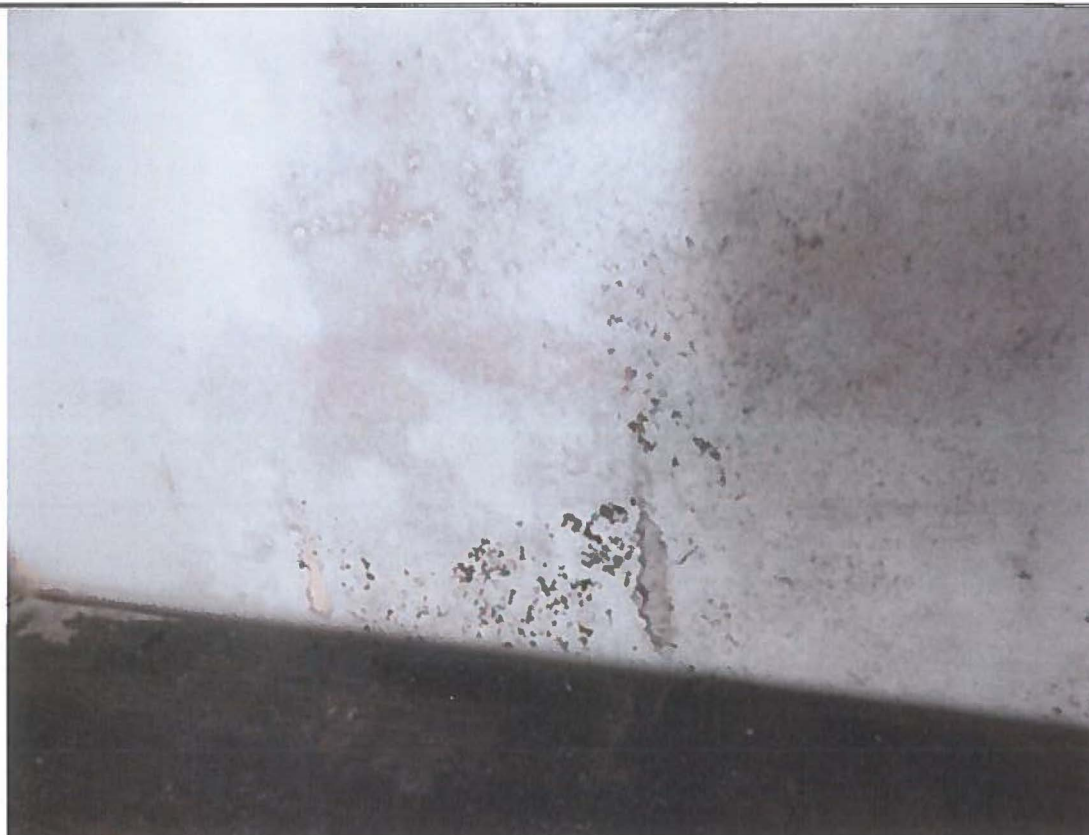
3 rd Floor – Suspect visible mold growth on west plaster wall in Command Center office.
