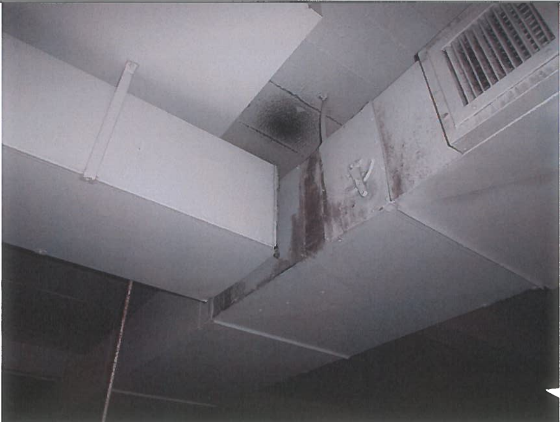
2 nd Floor – Particulate dust buildup in HVAC system (vents and diffusers) within the Fire Department area.
