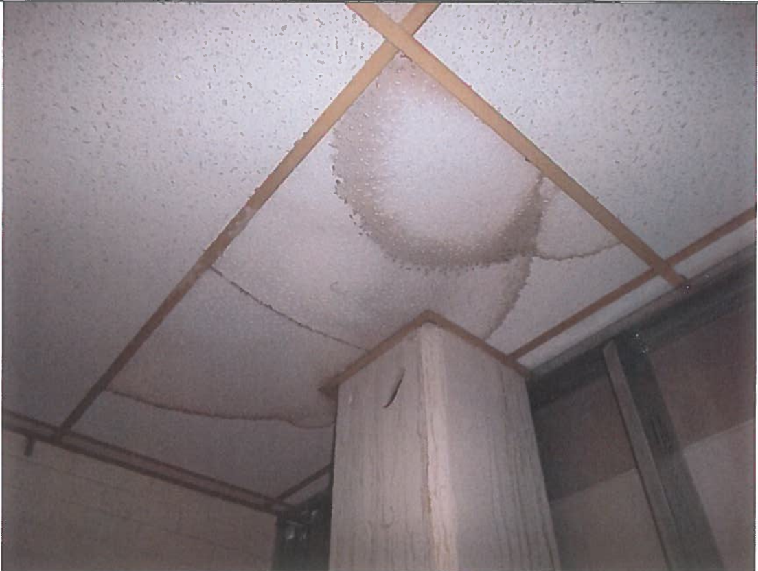
2 nd Floor -- Water staining on ceiling tiles and on column within the closet of the Detective's Office.
