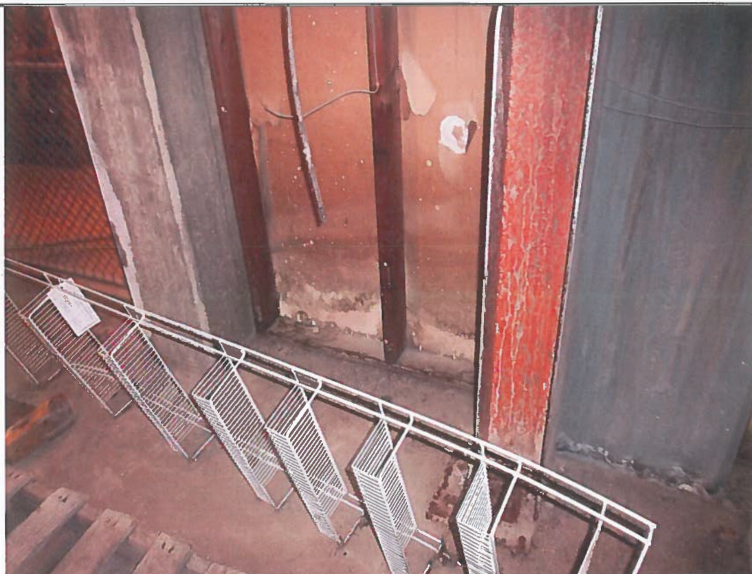
Basement – Water staining on west drywall wall of Bike Storage/Evidence Room.
