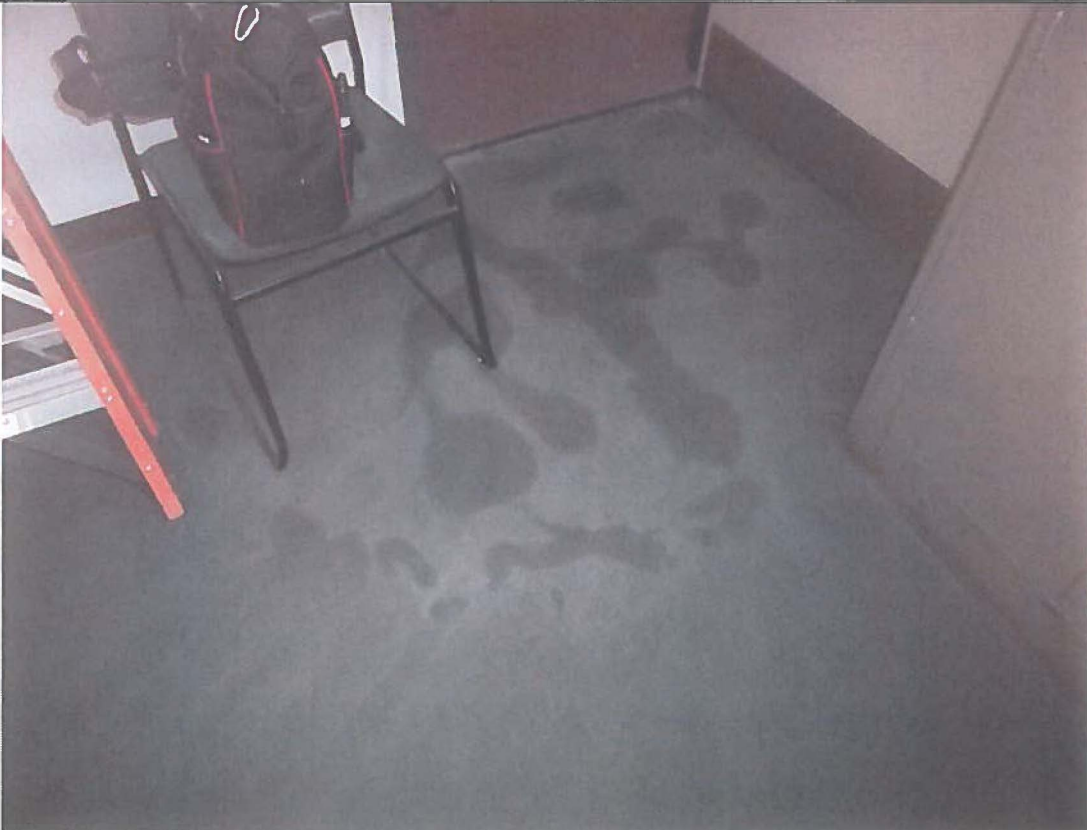
2 nd Floor – Saturated carpet (water coming from above ceiling) in foyer outside door of Fire Department.
