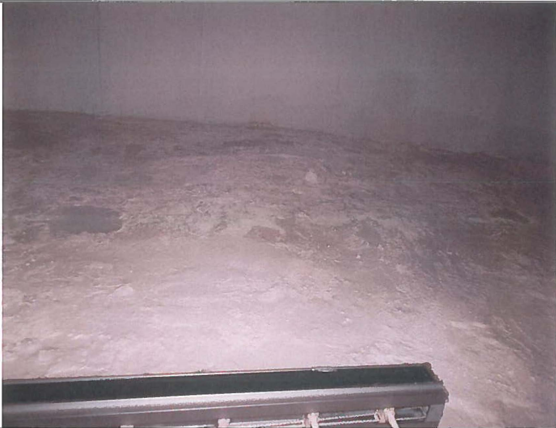
2 nd Floor – Water damage on east plaster wall and ceiling of Fire Department.
