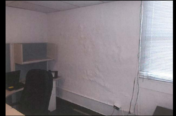
3 RD FLOOR – WATER DAMAGE EAST PLASTER WALL IN D.A.R.E. OFFICE
