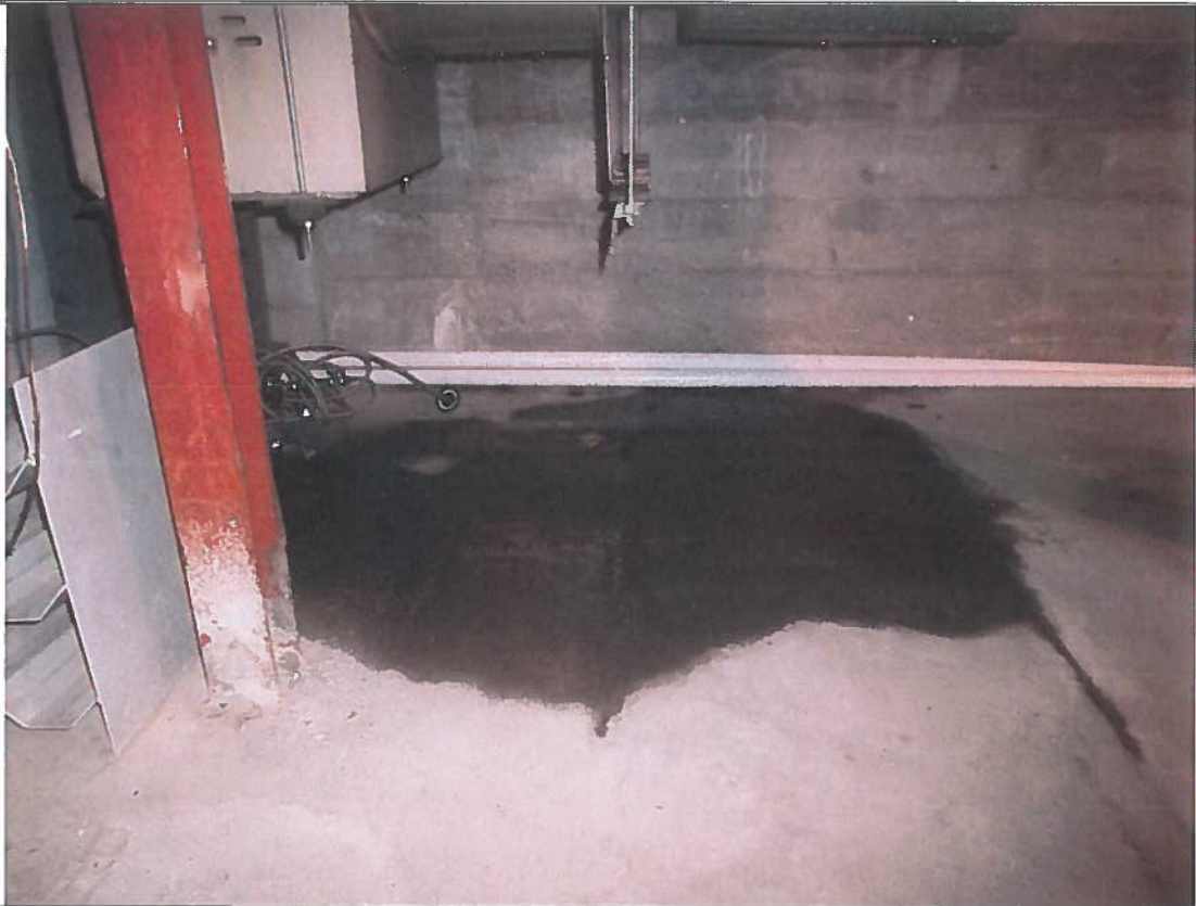
Basement - Standing water on concrete floor in Fire Department Storage area.
