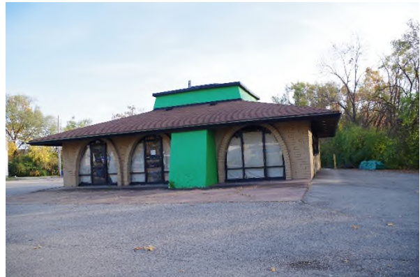
Deteriorated, vacant commercial restaurant building.
