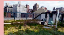
A green roof that limits runoff
