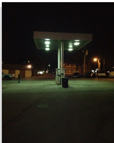
4 x 400 watt Metal Halide fixtures
