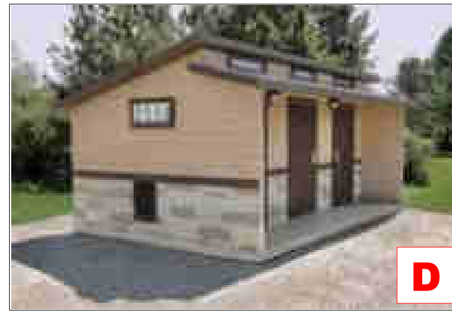
PRE-FAB RESTROOM BUILDING W/STORAGE
